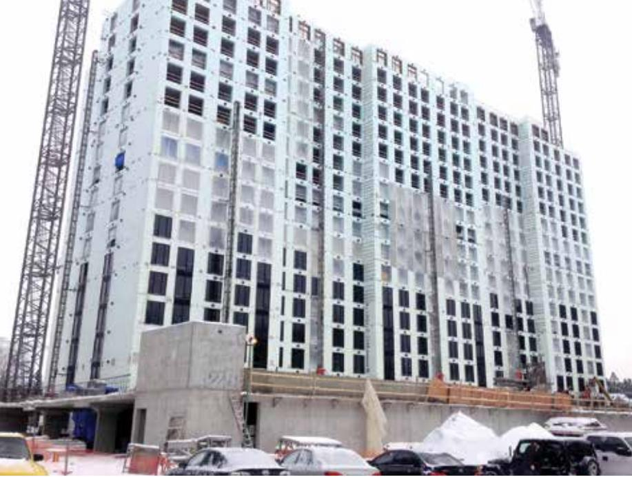
This project has pushed the known boundaries of ICF in high-rise buildings – for example, techniques to use ICF in stairwells, elevator shafts and other areas that require modification or removal of the foam needed to satisfy relevant building codes. These efforts were made due to the high speed of installation and inherent cost savings over traditional builds. ■
